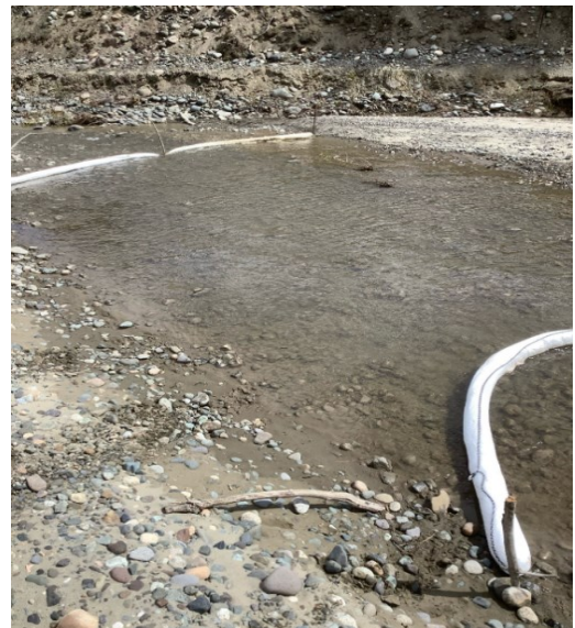
EM recommended that stream/wetted soil crossing with quad should have spill containment in place. Crews placed a spill barrier on both sides of crossing.
